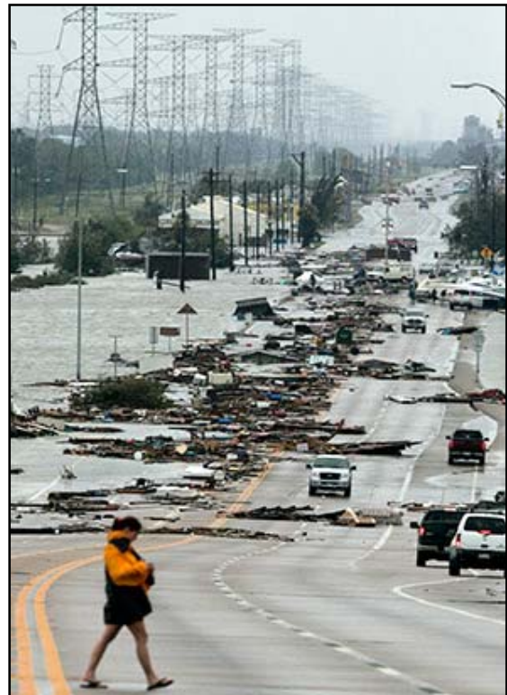
Figure 30. Debris on SH 146 in Kemah and Seabrook, 9/13/2008 (ABC News)
