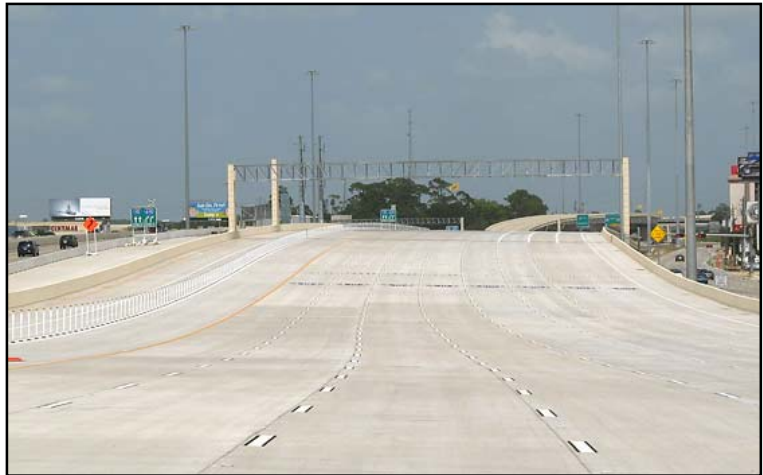
Figure 4. IH-10 (Katy Freeway) West of IH-610 Before Grand Re-Opening, July 2008
